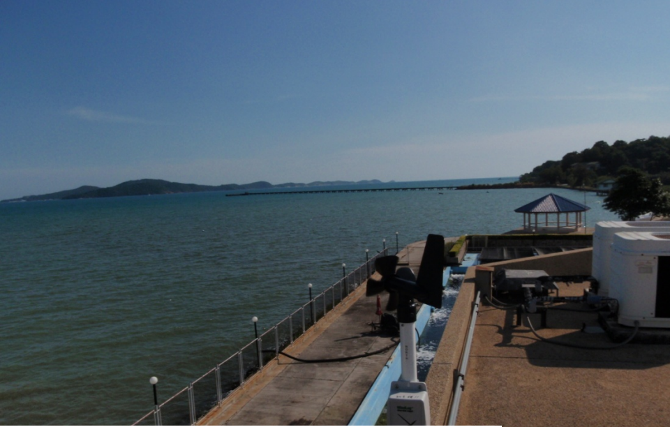
EMDEC Aquarium roof
